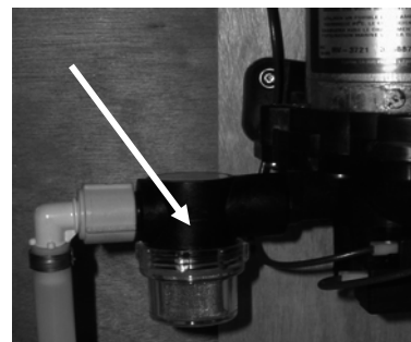
Fig. 7.2 Water pump strainer
